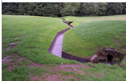
The completed ditch, 13 th hole on the Hilton
